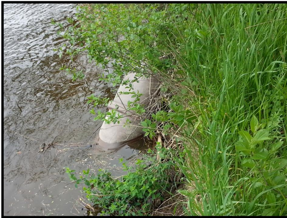
**Figure 5:** 20SA722, eroded well casing.
